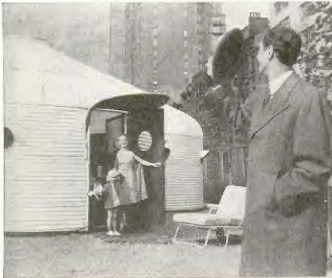
It takes only a few hours to erect this "igloo" of corrugated metal. Diagram shows floor plans
